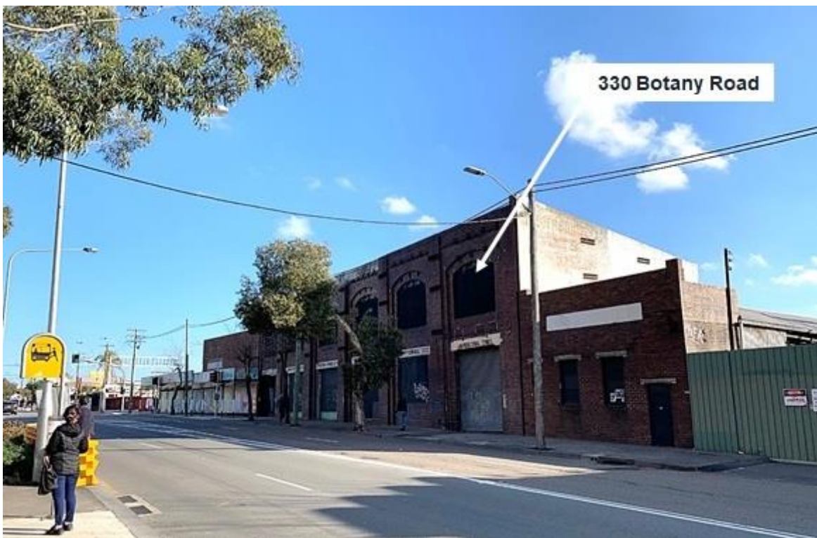
Figure 4: City owned properties adjacent to the south at 330 Botany Road.
