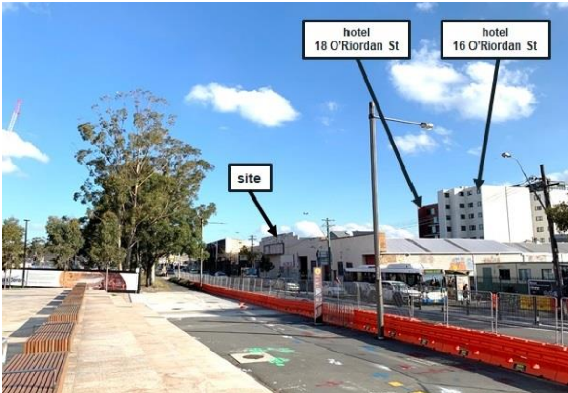
Figure 5: View to the site from Green Square Plaza.
